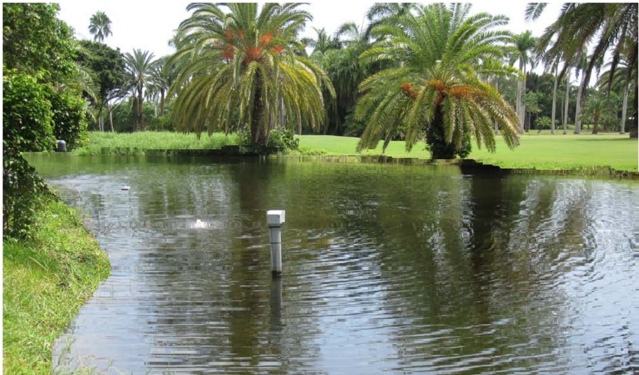
Figure 72. Aerated retention pond
