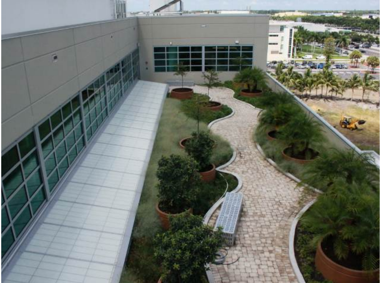
Figure 57. Photo of a green roof installation at FAU Engineering East in Boca Raton, FL
