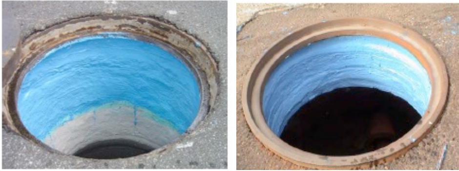
Figure 89. Chimney seal installed (Courtesy USSI)
