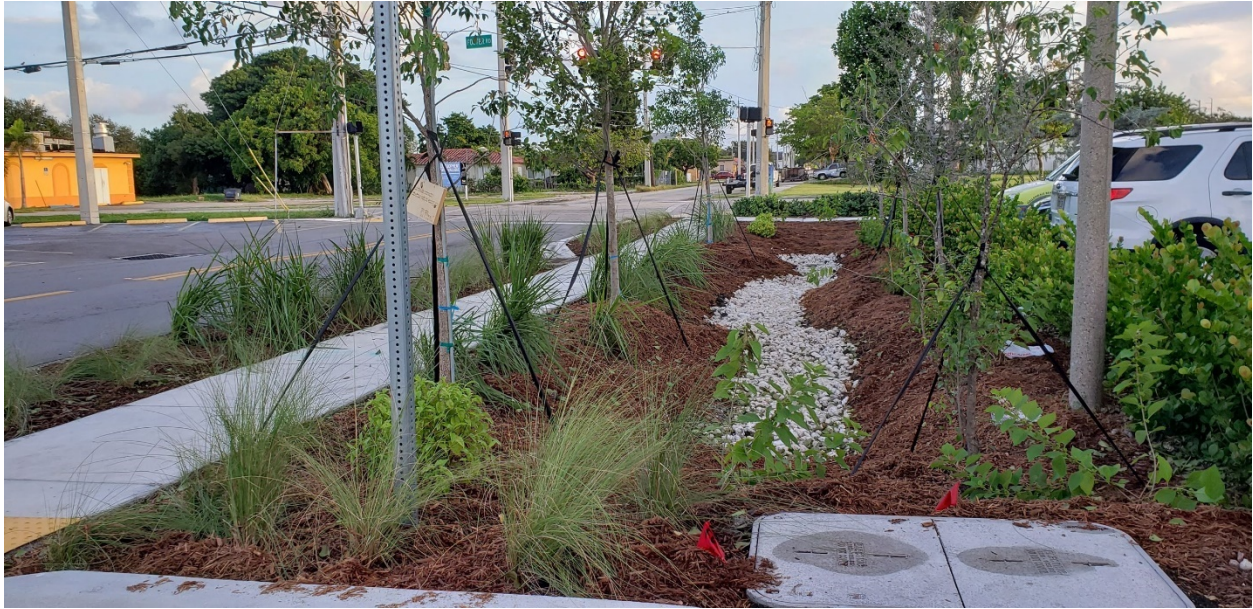
Figure 59. Photo of a bioswale pilot installation in Hallandale Beach, FL ( https://www.hallandalebeachfl.gov/ )
