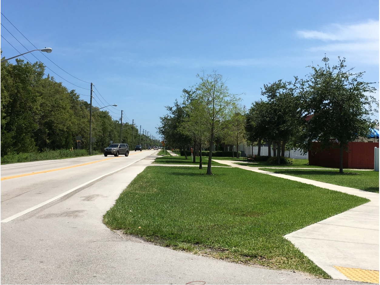
Figure 70. Roadway dry swale
