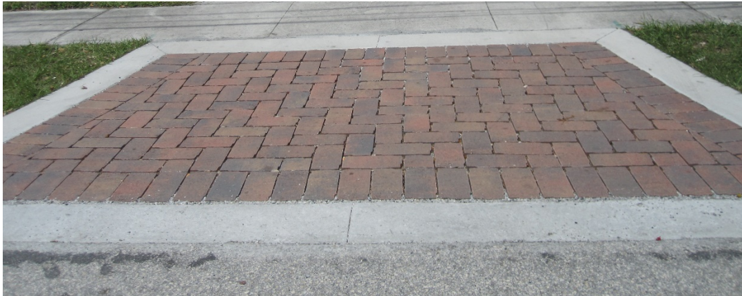
Figure 63. Example of a pervious paver driveway
